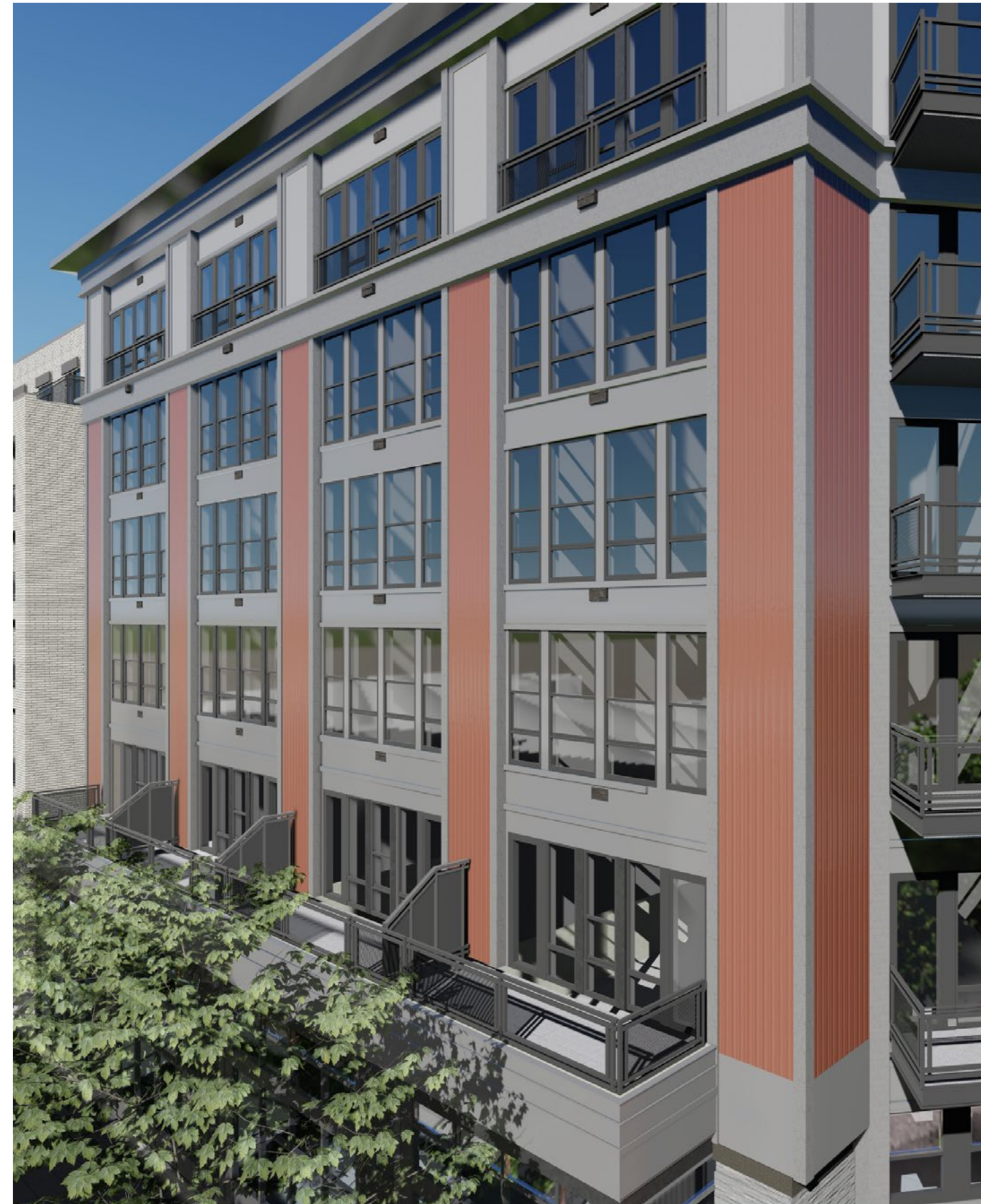
North Identity Balconies
